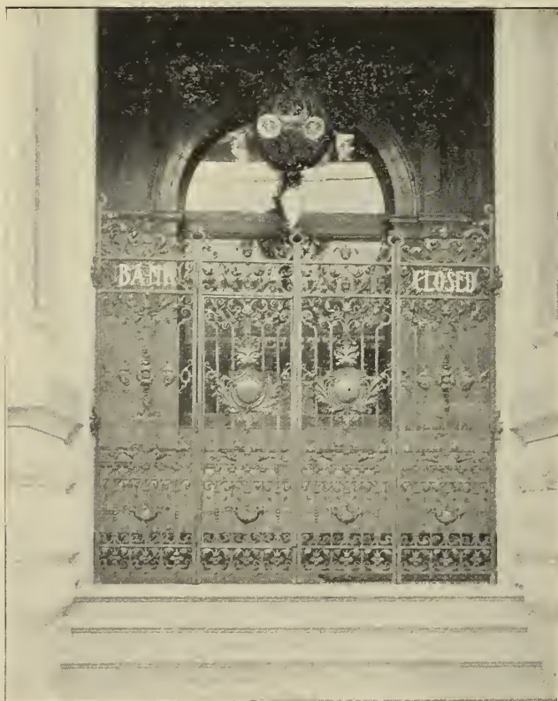
C.—ENTRANCE GATES, GERMAN BANK BUILDING, SAN FRANCISCO. Wrought Iron, Bower-Barffed.
